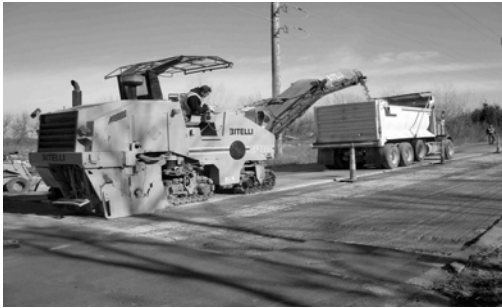
Mill and overlay = new asphalt
