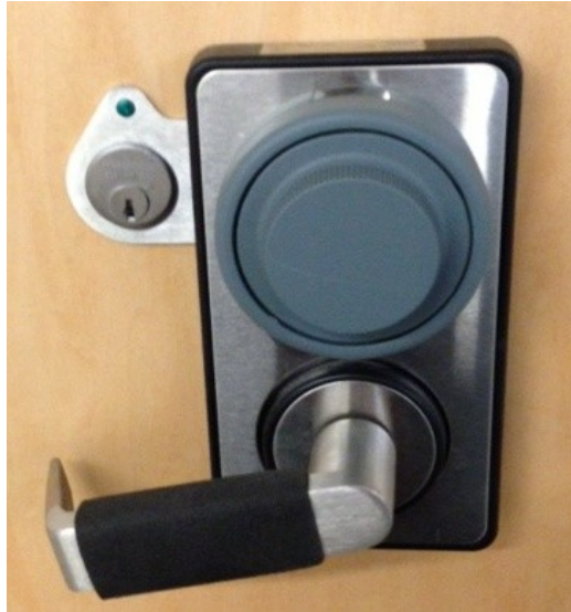
Figure 4-1 Combination door lock with bypass key lock
