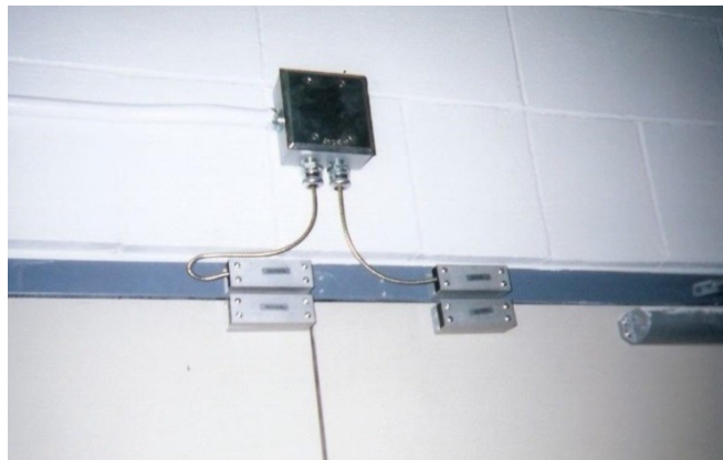
Figure 4-5 Triple-biased BMS sensor on double doors
