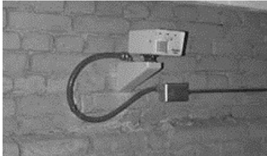
Figure 4-8 Dual technology sensor
