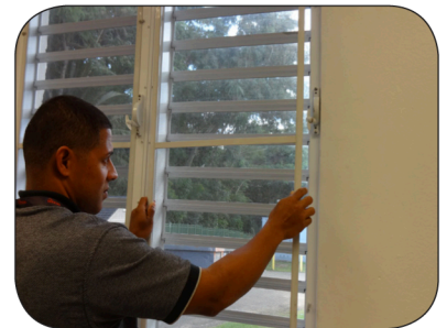
Install or repair window & door screens.
