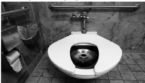
Replace wall mounted toilets for floor mounted
