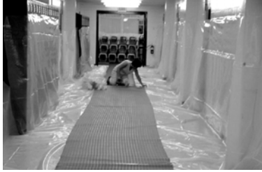
Placing rubber runner
