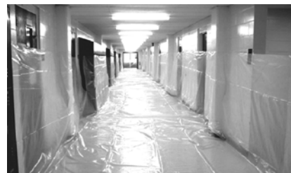
Lining hallway with plastic
